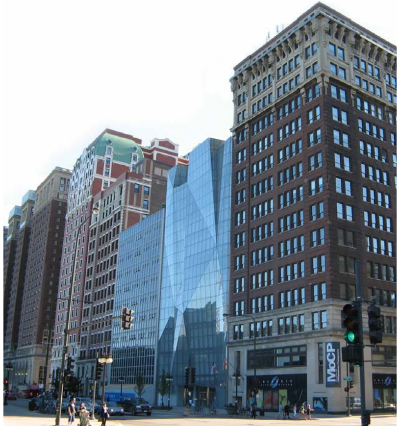
View from Michigan Ave.
