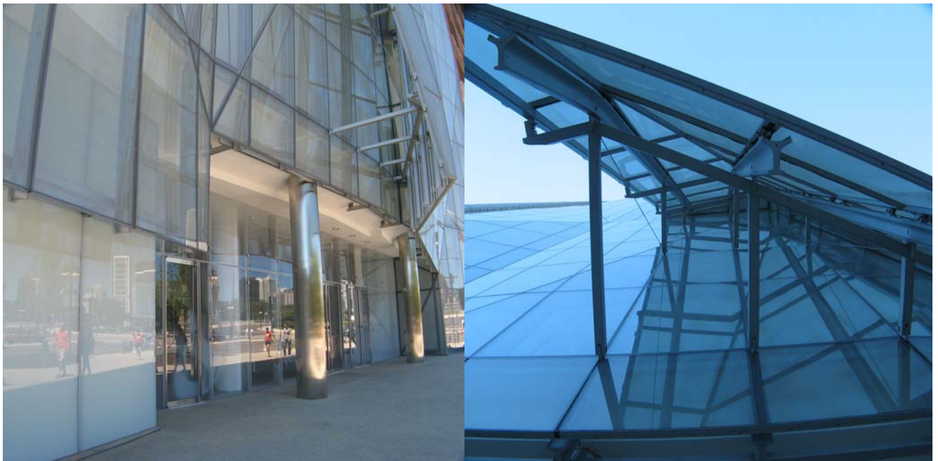
Image 1 – Building Entry and Canopy
