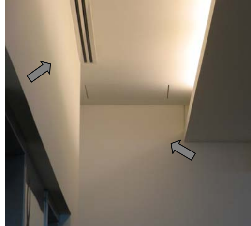
Image 3 – Spill light from Elevator cove
